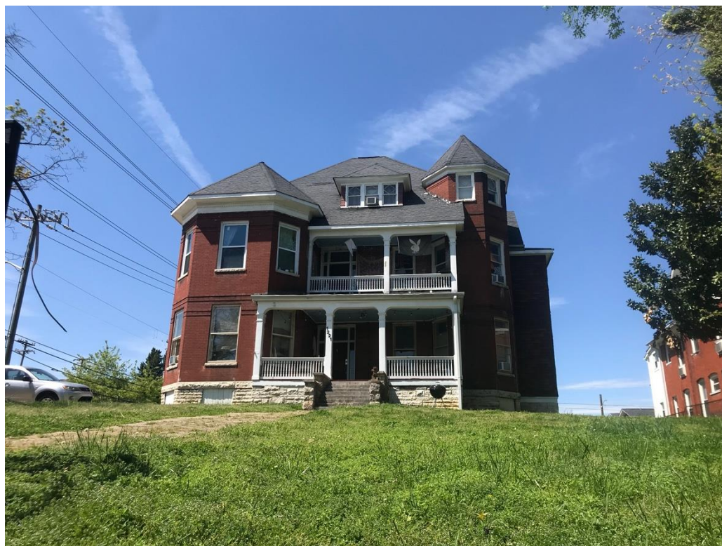
Figure 2: Historic home in Fort Sanders. Source: Yael Uziel
